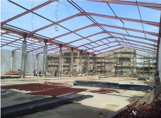
Erection of steel Trusses and roofing-Meera Investments Ltd
