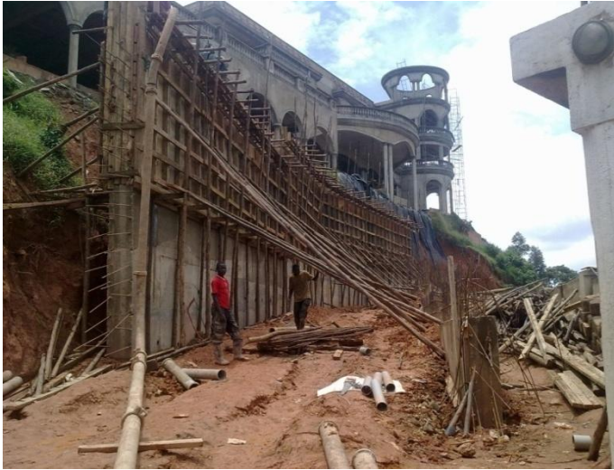
Casting of RCC Retaining Wall and Foundation Steel Works
